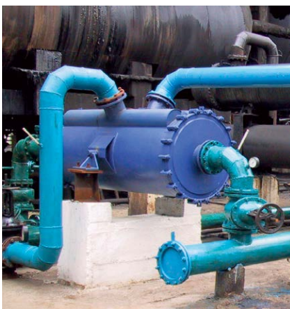
Alfa Laval spiral heat exchanger used as BO/DBO interchanger at Avdeevka, Ukraine
