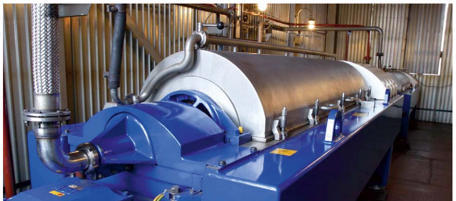
OA0 Koks uses two Alfa Laval decanter centrifuges for coal tar cleaning at its Kemerovo plant
